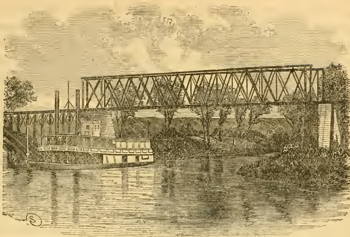
N. P. R. R. BRIDGE OVER MISSISSIPPI, NEAR BRAINERD, MINN.
